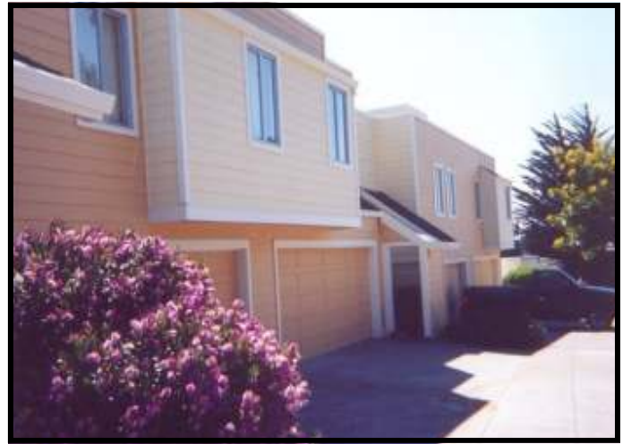
View of completed garage repairs
